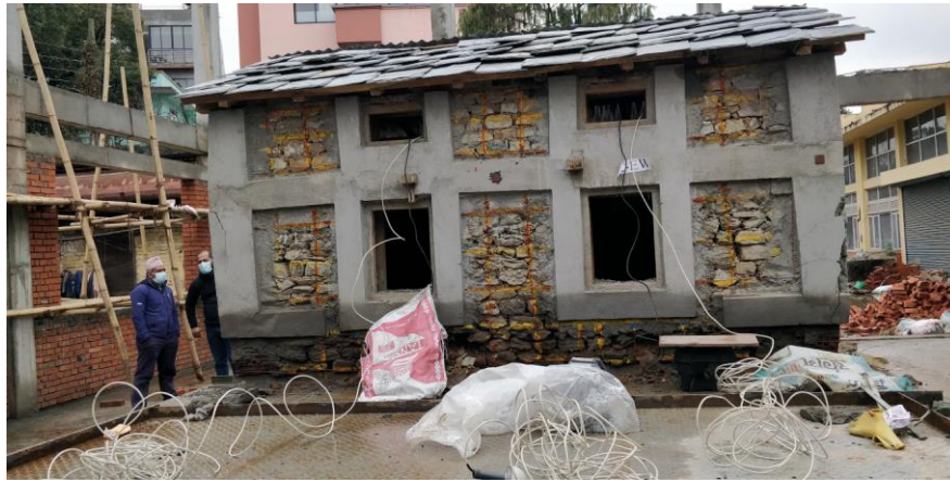
Figure 1: Instrumentation for vibration recording.
