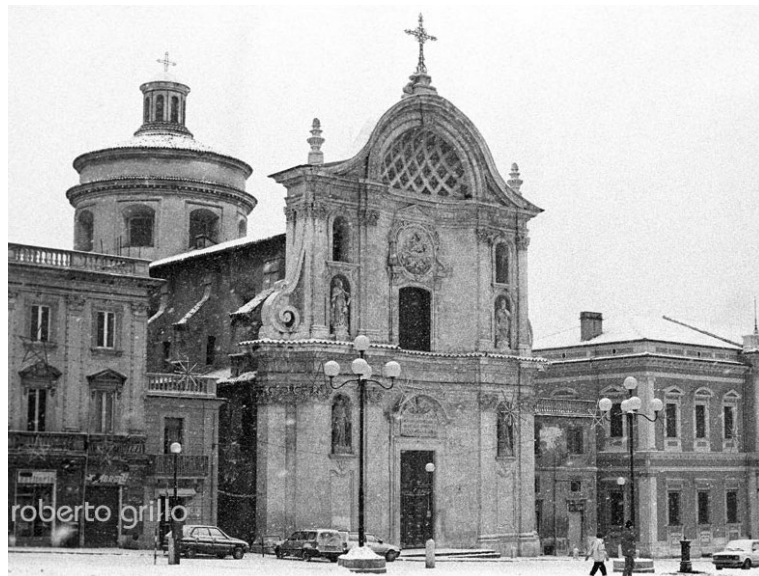
Figure 1. External view of Church of Santa Maria del Suffragio. From the cathedral square in L'Aquila.
