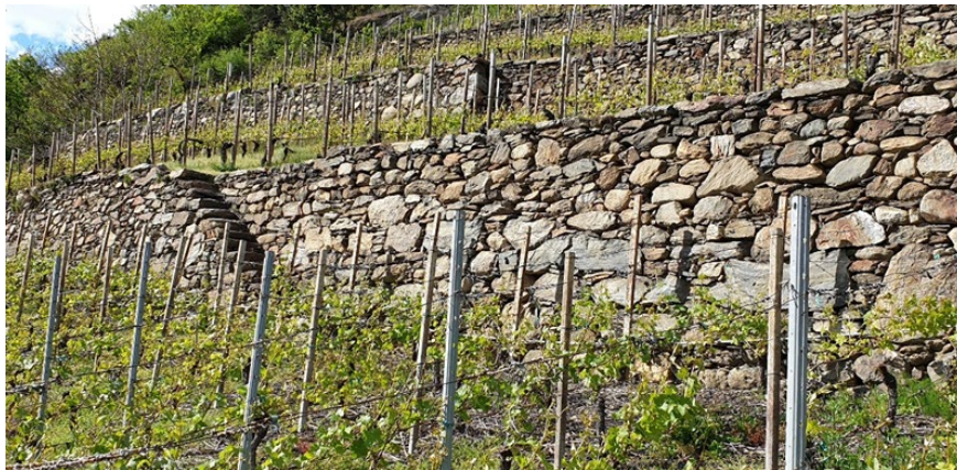
Figure 2: Typical facing of a drystone wall of the Valtellina terraces
