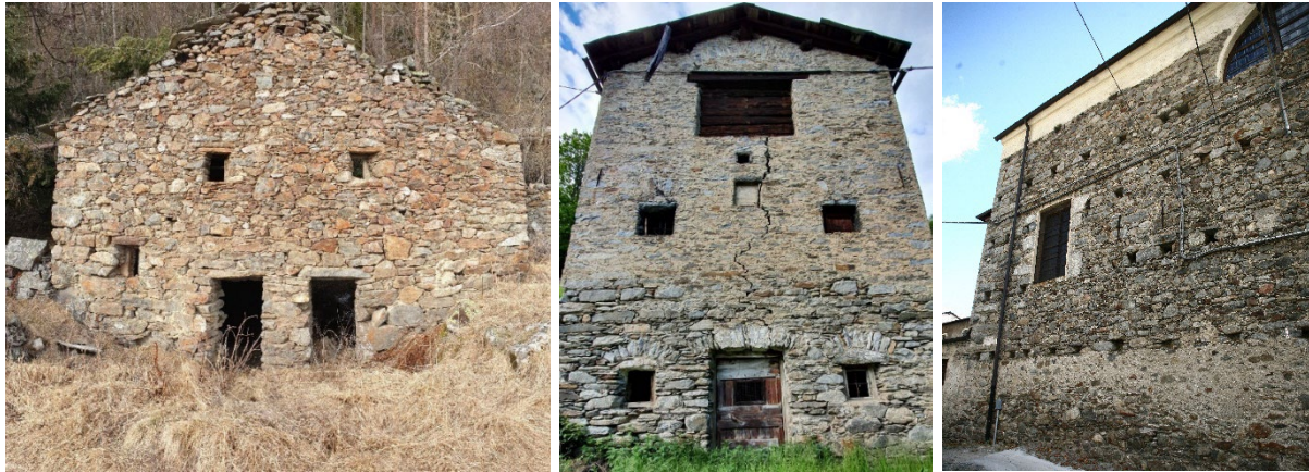
Figure 3: Similarities among the drystone rural construction (left), stone and mortar rural construction (middle) and stone and mortar wall of the church of S. Ignazio in Ponte in Valtellina (right)
