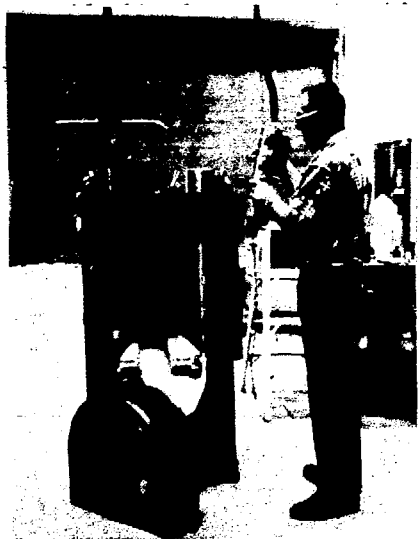
FIG. 6 - ASSEMBLY OF THE 18-inch FAST-CLOSING GATE-VALVE.
