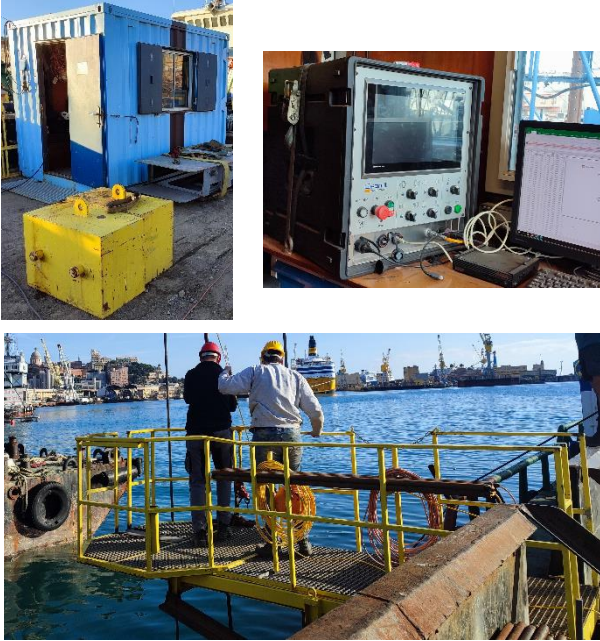
Figure 4. OFFICE CONTAINER, MANTA CONTROL UNIT AND CANTILEVER
