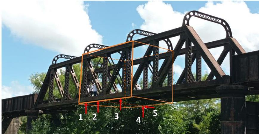
Figure 9: Santa Lucía Bridge with the location of the sensors and orientation of its axis – Bridge test.
