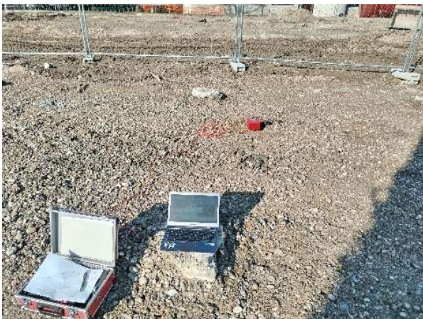
Figure 9. (HVS3) tests after the construction of the piles
