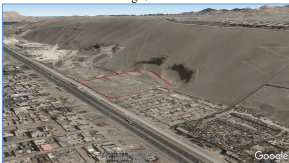
Figure 3. 3D image (looking NE) of the project site. The extent of the site is indicated with a red polygon. North side of the site along the toe of Lomo Corvina (Google Earth image).
