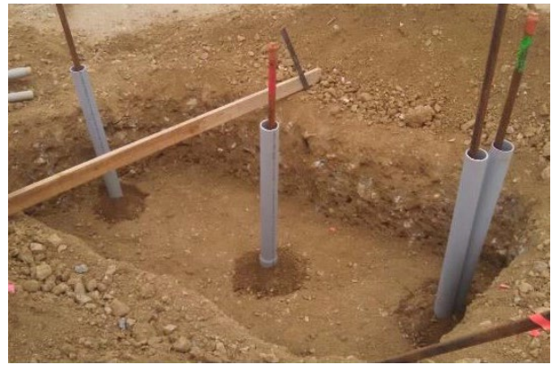
Figure 5. Final Installation of Settlement Monument (SM) 15
