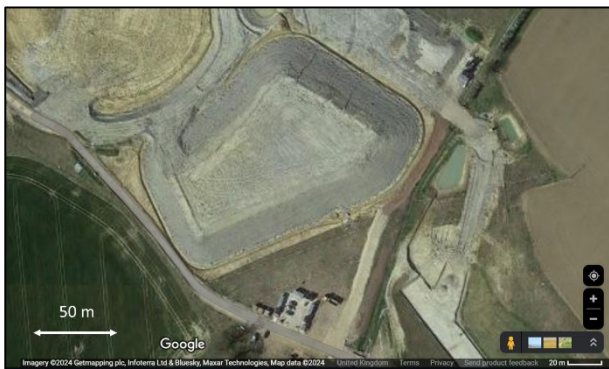
Figure 2. Aerial photo of the 8.2 m high trial embankment (Image courtesy of getmapping plc, Infoterra Ltd & Bluesky, Maxar Technologies, Mapdata @2024)
