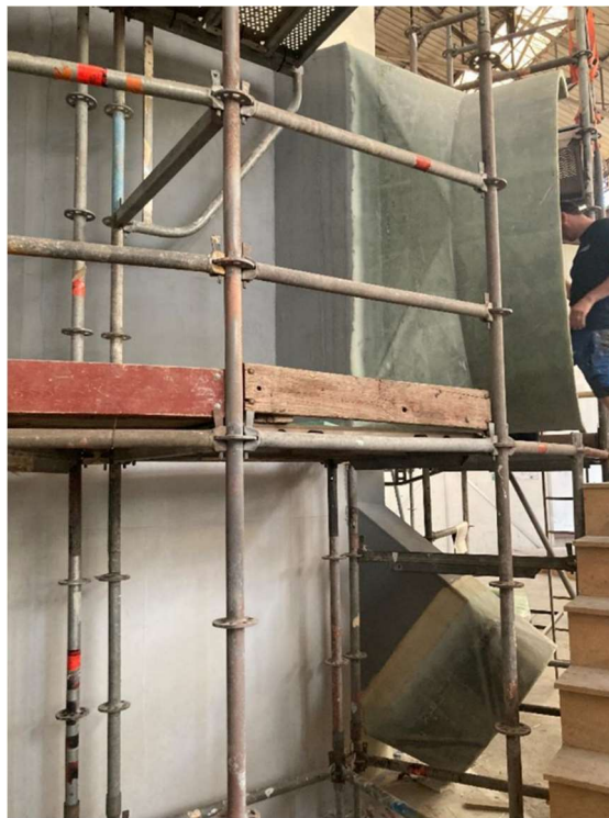
Figure 17 : Tubes connected to module D
