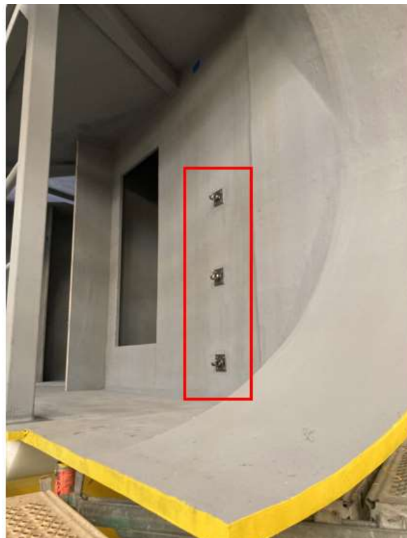
Figure 19 : pad eyes for safety line
