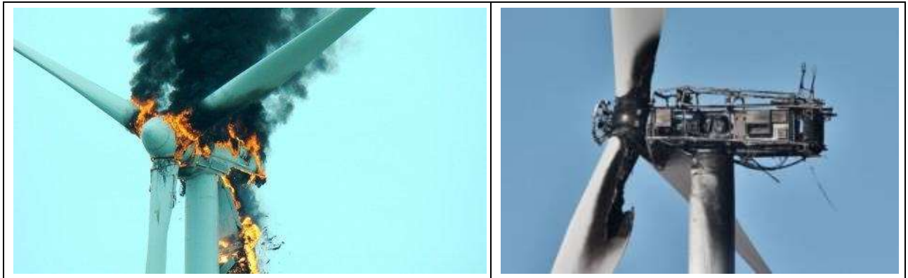
Figure 7: Fire accident in onshore wind turbine (17)
