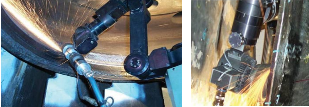
Figure 2: The configuration of the SCOMPI robot during the grinding process
