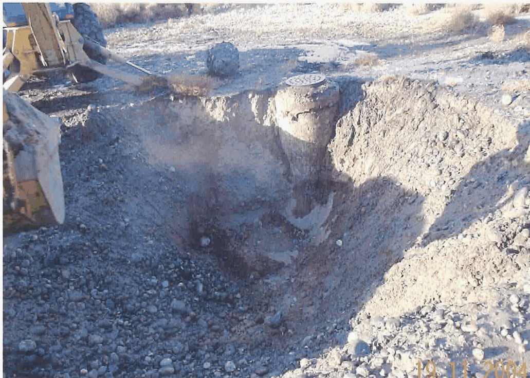
Figure 5. 100-F-26:10 Pipeline Subsite – Service Area 1, Stake Number 39 Test Pit.
