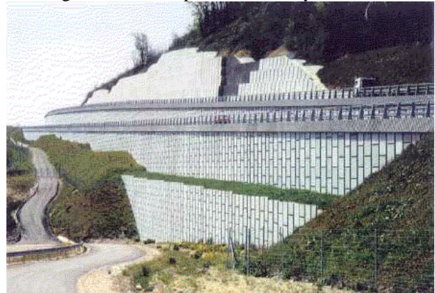
Figure 4: Tèche retaining structure ((Monnet and Allagnat 2001))
