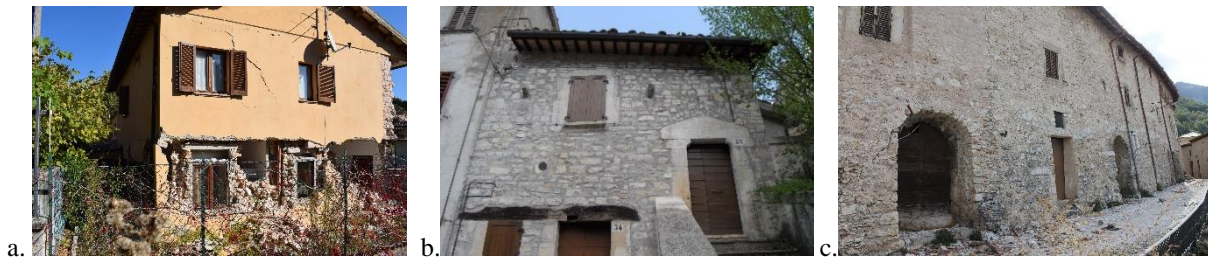
Figure 5: a) Class A building: poor masonry quality and floors replaced with rigid ones (MCC); b) C class building: random layout limestone masonry reinforced by deep repointing with cementitious mortar (CSN); c) D class building: random layout limestone masonry reinforced by grout injections and r.c. jacketing (internal side) (CMP)
