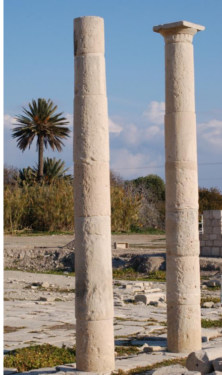
Figure 1: Ancient free standalone multi-drum columns (Amathus, Cyprus).
