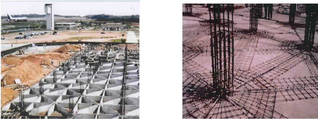
Figure 8. The shallow foundation system called SNSF
