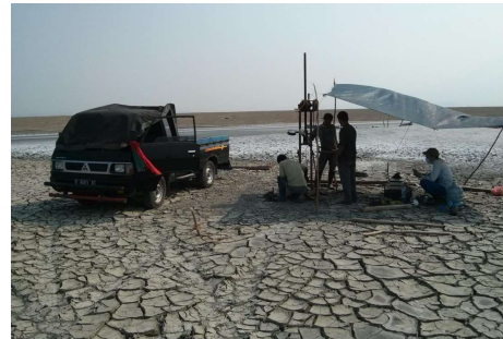
Figure 19. The geotechnical team conducted CPTu 9 inside mud area at elevation +9 m
