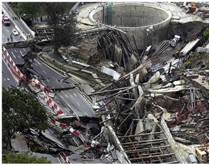
Figure 3. One of the cause of Nicol Highway Accident in 2004 is due to the existing residual excess pore pressure
