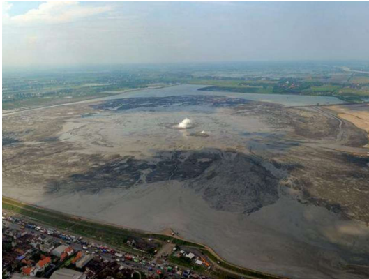
Figure 16. Situation of the mud surrounded by defence dykes and the traffic nearby, this photograph was taken in 2009
