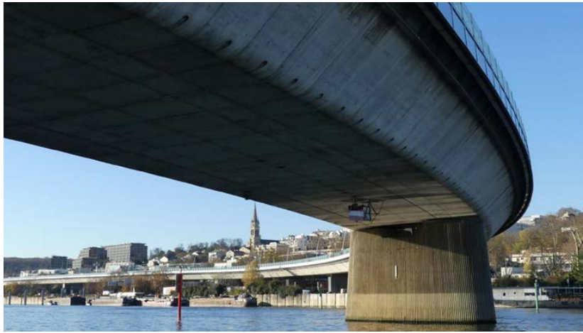
Figure 1. Picture of the Saint-Cloud Viaduct (Saint-Cloud city in the background).
