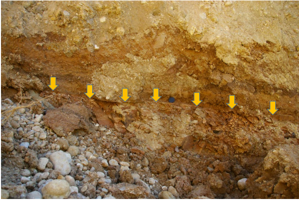
Figure 5. Shearing surface visible in an excavated face.
