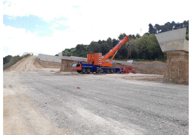
Figure 7. Construction of the piles loading platforms and box girder beams.
