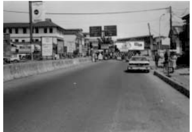
Photo 2 Spoilt traffic light, absence of road marking, and obsolete concrete road partition which is not crash-worthy
