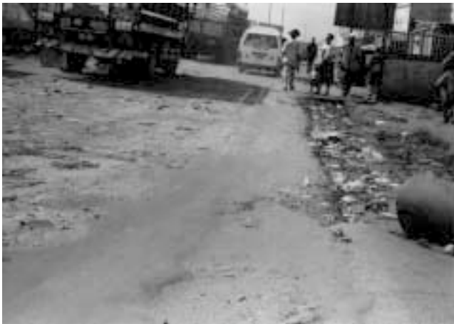
Photo 1 Rough road surface, blocked drainage with pedestrian walking side by side with the vehicular traffic
