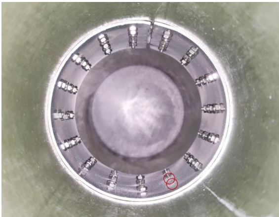
Figure 125 – Post-testing inspection from the inside (specimen #2)
