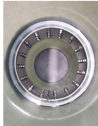
Figure 90 – Interior of the GFRP tubes after bolting
