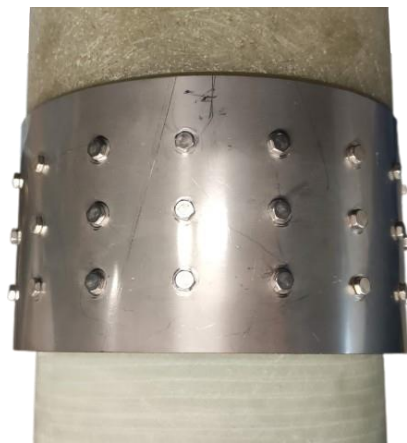
Figure 108 – Post-testing inspection from the outside (specimen #1)
