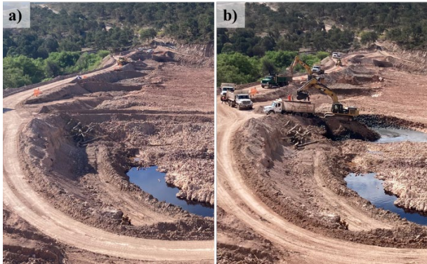
Figure 17. a) Excavation stopped at ~1880 m, b) Excavation during stage 6 below 1879 m.
