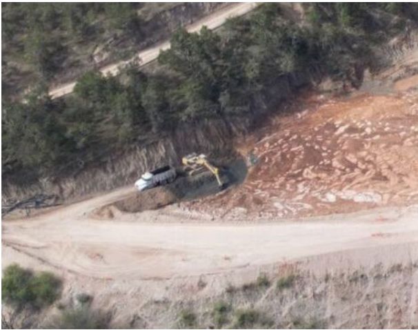
Figure 13. Excavation point in the south margin (stage 3).
