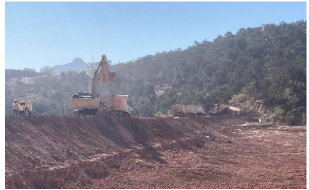
Figure 15. CPT-Pond-04 excavation area near the dam embankment.
