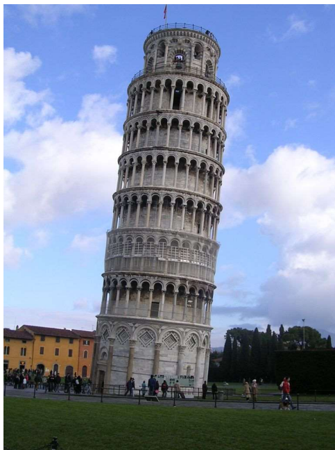
Figure 1. The Leaning Tower of Pisa.
