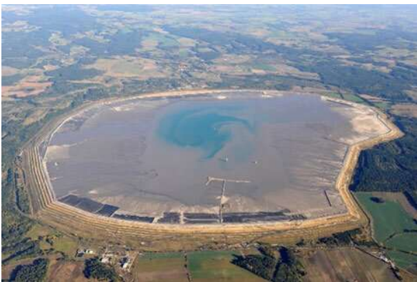
Figure 7. Zelasny Most tailing dam (Poland).
