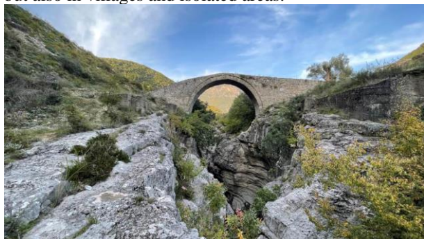
Figure 1. “Brari Bridge”, Tirana.
