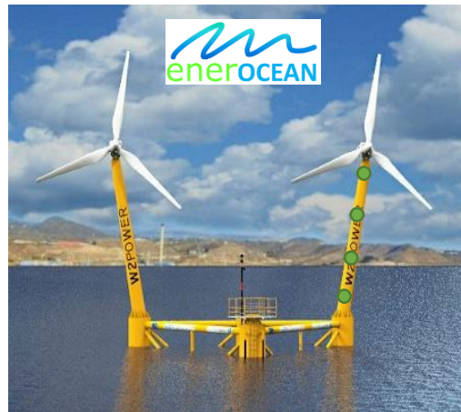
Figure 2: SHM of W2Power tower - 4 levels distribution.
