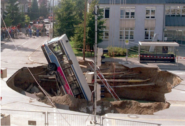
Figure 2. A sinkhole swallowing a bus (source: picture-alliance/dpa)
