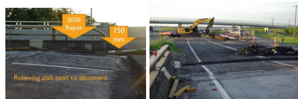
Figure 8. 2020 releveling of 1991 adjacent bridge with 150mm drop in the relieving slab
