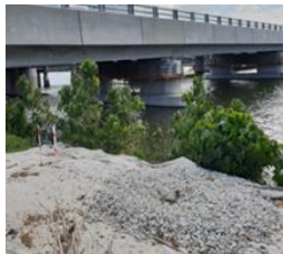
Figure 17. Gravel back fill placed at OSP4B
