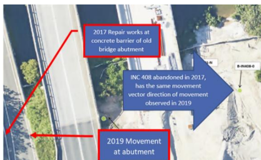
Figure 6. Repair works undertaken
