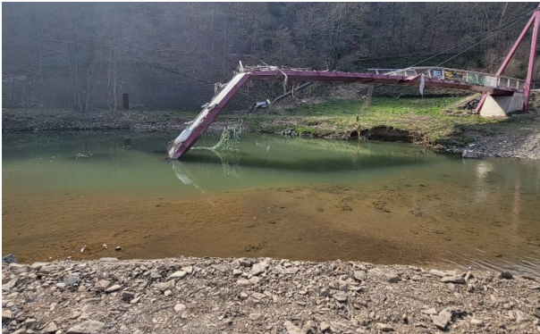
Figure 1. Pink pedestrian bridge in Mayschoss, Germany after the July 2021 western European flood event.
