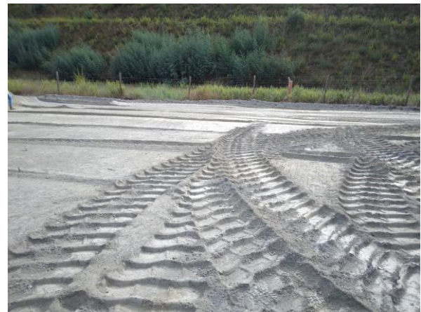
Figure 4. Black schists in the earthfill.
