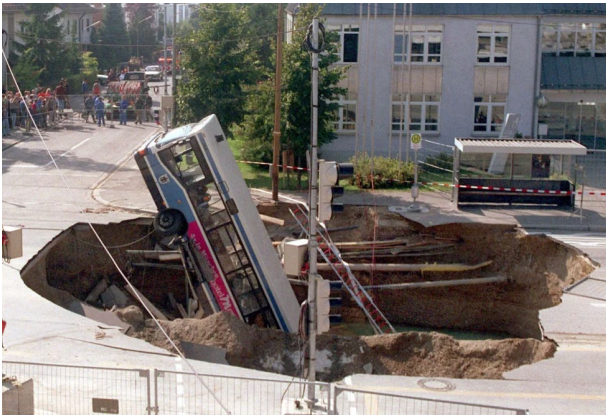
Figure 2. A sinkhole swallowing a bus (source: picture-alliance/dpa)
