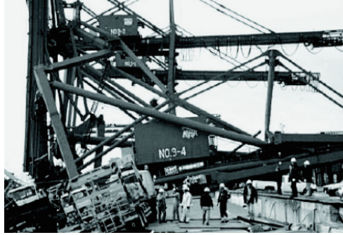
Fig. 1: Collapsed cranes after the Kobe Earthquake [2]
