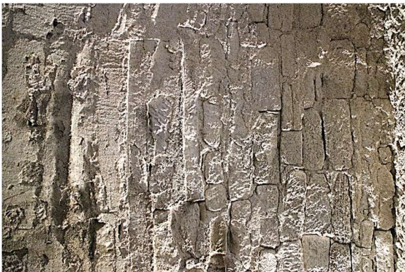
Figure 9: Vault cover of the lower floor
