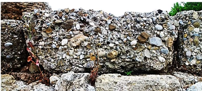
Figure 3: Example of conglomerate block used in foundations
