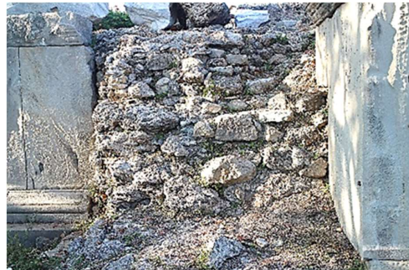
Figure 10: Infrastructure of one of the side stairs
