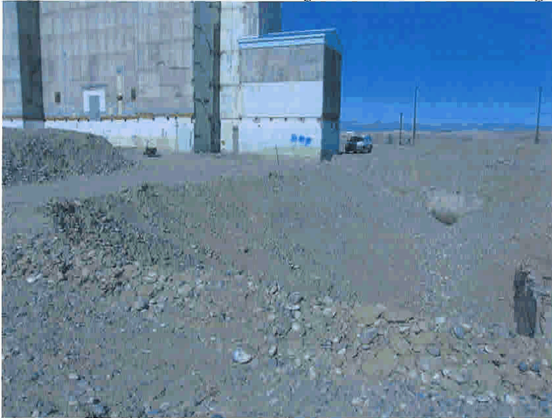
Figure 8. 100-F-26:15 Excavation Looking North to 105-F Reactor Building.
