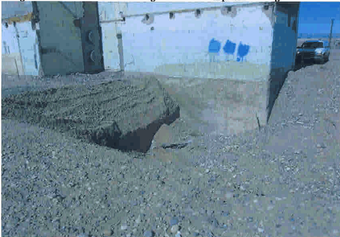
Figure 9. 105-F Reactor Building Foundation Exposed During Excavation.
