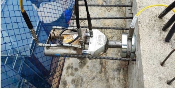
Figure 2. Control of post-tensioning works in a concrete slab during building construction.
