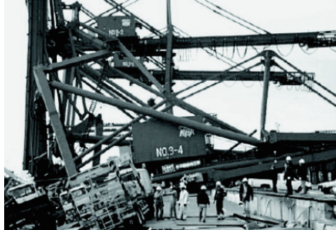
Fig. 1: Collapsed cranes after the Kobe Earthquake [2]
