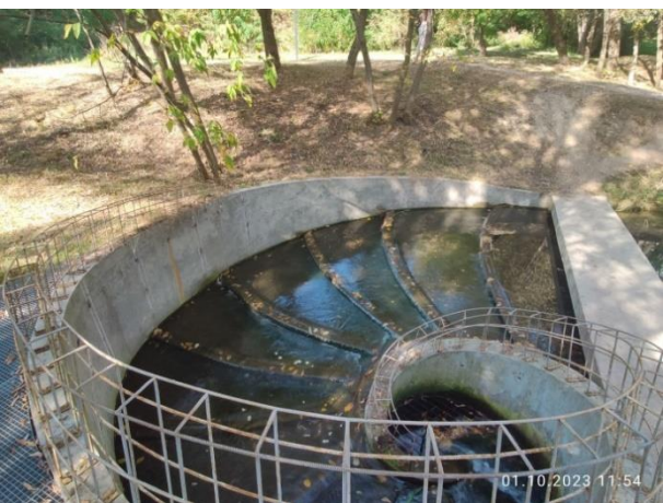
Figure 5. Artificial islands and snail-shaped spillway
